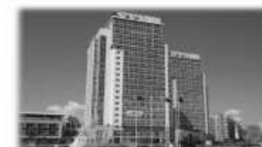
HOUSING PROJECTS IN Khabarovsk (Kyeryong Construction Industrial Co., Ltd., Republic Of Korea)
